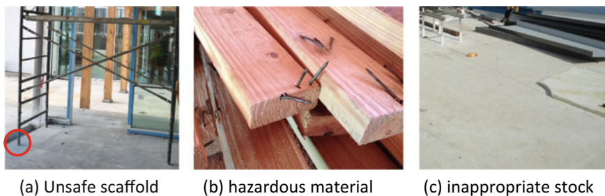
Fig. 135.5 On-site issues requiring preventive actions
