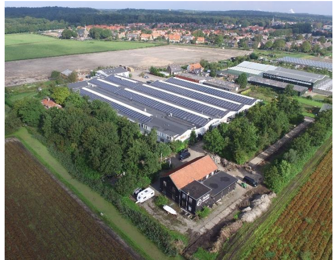
Figure 7: The roof of the Fablo tennis court
