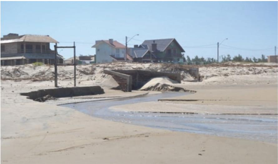
**Fig. 3.7** Erosion caused by the southward displacement of the washout's mouth
