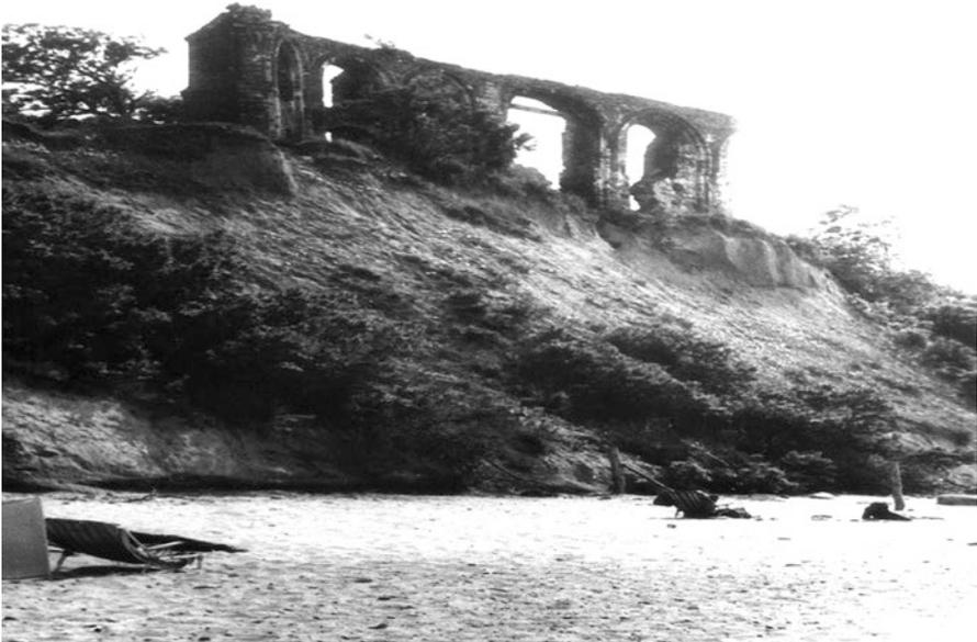
**Fig. 6.17** The north-eastern fragment of the Trzęsacz church in 1976. Visible in the cliff glacial tills, as a result of sea waves action move down towards the beach
