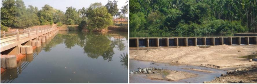
**Fig. 21.7** Sediment trapping by the vented dams constructed across the rivers which otherwise would have reached the near shore and finally added to the beaches
