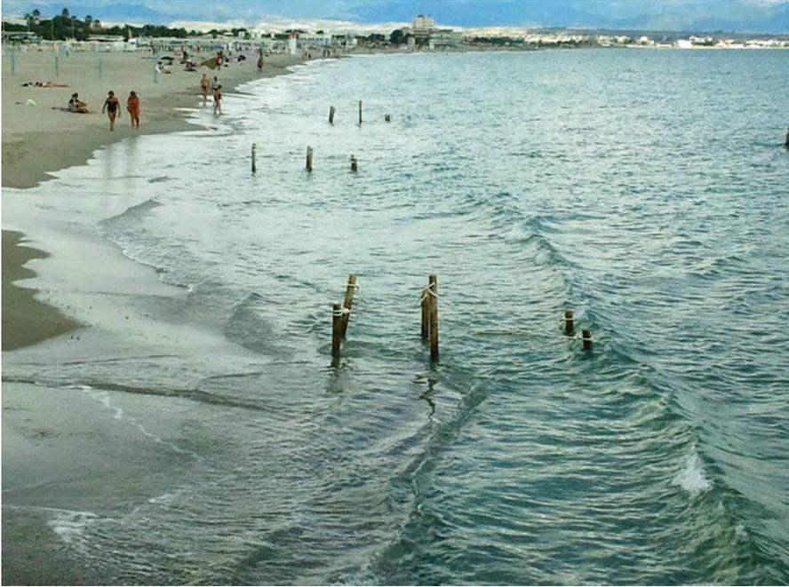
**Fig. 15.7** Rope railings to assist people to cross the step on the Poetto beach (Cagliari, Italy), where the profile was milder before a nourishment carried out with coarser sediments
