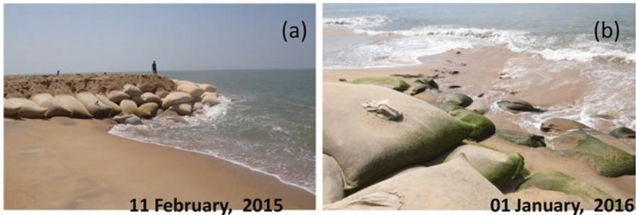
**Fig. 21.6** Geo-textile reefs are also in dilapidated conditions at Ullal-Kotepura Beaches during installation (a), and just about a year later (b)
