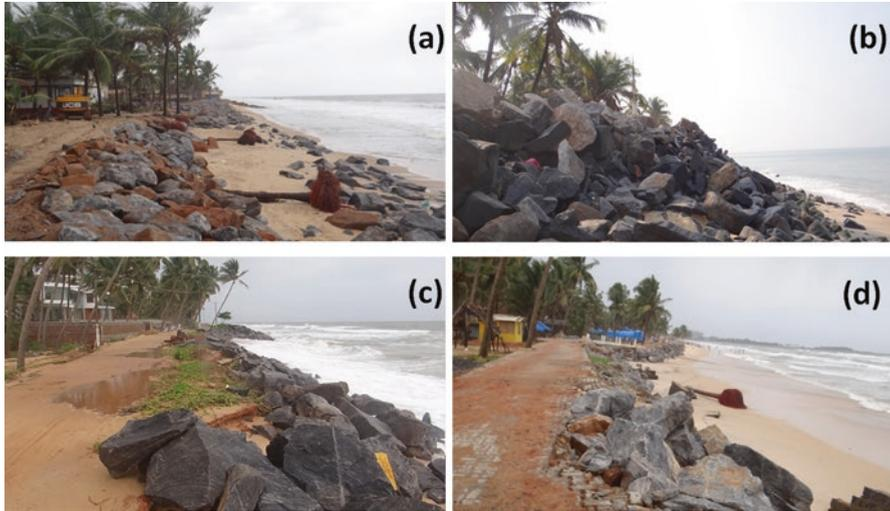
**Fig. 21.3** Failure of seawalls at Talapady (a), Ullal (b), Udyavara (c), and Malpe Beaches (d)
