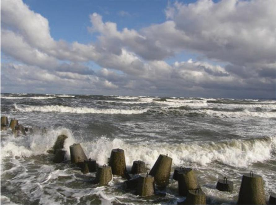
**Fig. 6.22** Tetrapods protecting the eastern harbour breakwater in Świnoujście (Source: Google Earth-Image-2016 CNES/Astrium-Date 5/2/2016)
