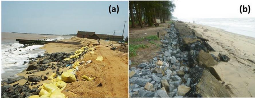
**Fig. 21.5** Destroyed seawall & sand bags (a), and gabion retaining wall (b) at severely eroding Ullal-Kotepura beaches
